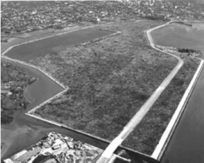
The CSCRP envisions to create 330.9 ha. of additional land for industrial and export processing use.
