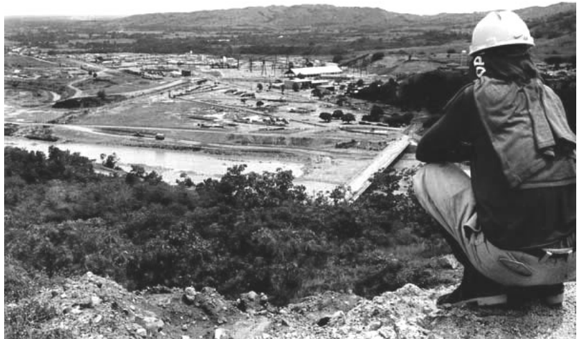
San Roque Dam, a $1.19 billion project funded by JBIC, is implemented by a consortium of foreign corporations led by Marubeni
